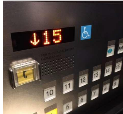
Emergency call in the elevator
