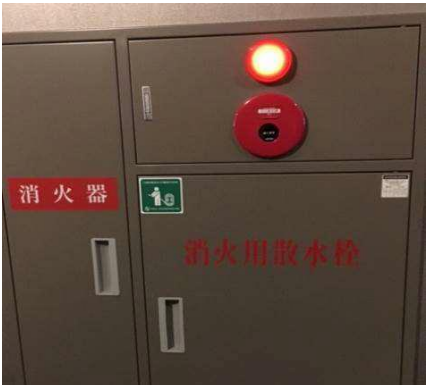
Fire extinguisher, Emergency Button, and fire hydrant in The corridor
