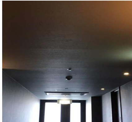
Fire alert, sprinkler and smoke detector in the corridor
